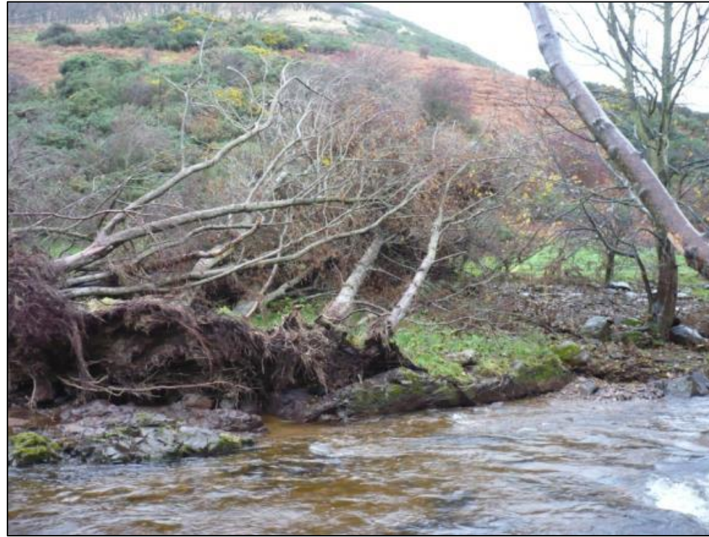
Flooding and bank erosion
